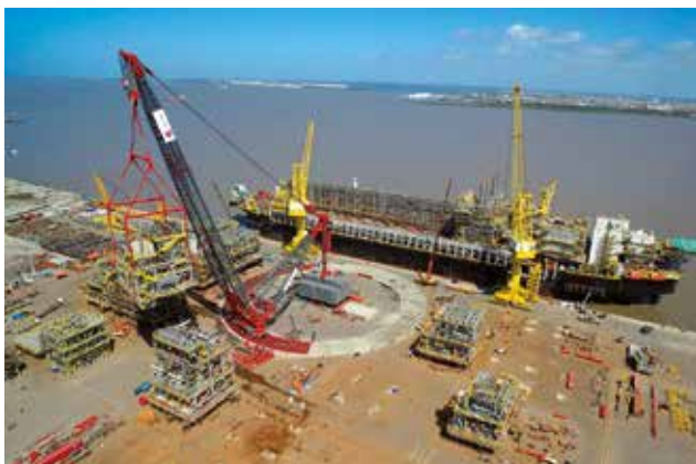
ALE mobile crane
